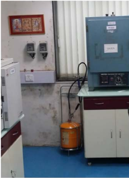
NASA 100MMT for fire safety of an electrical research laboratory
