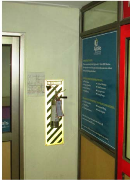
non magnetic NASA 227 MAR installed for fire safety of MRI machine at a hospital
