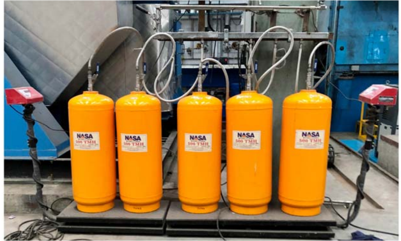
Typical NASA fire suppression system installation
